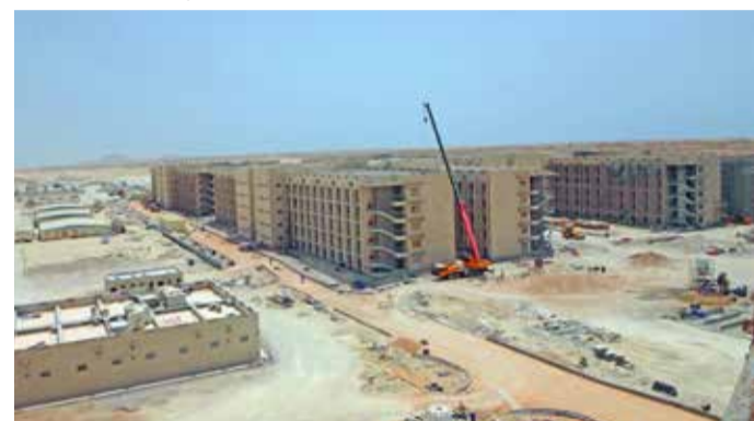
Progress at the flagship Renaissance Village in Duqm
