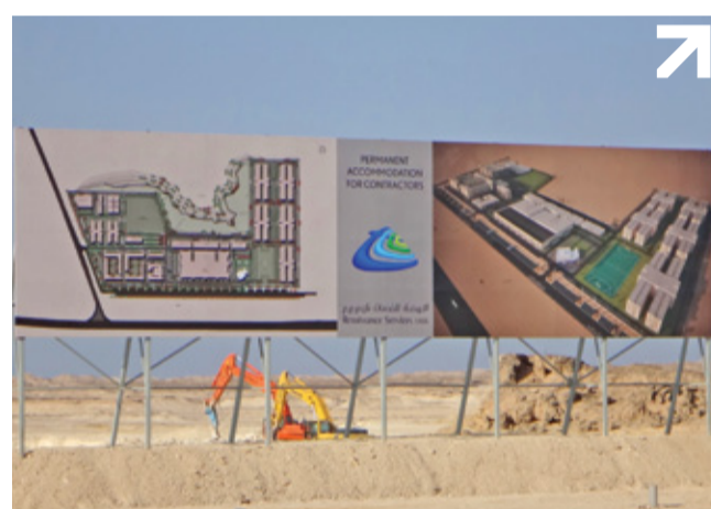
RS CSG's Permanent Accommodation for Contractors (PAC) development project at Duqm will accommodate 16,000 personnel when complete.
